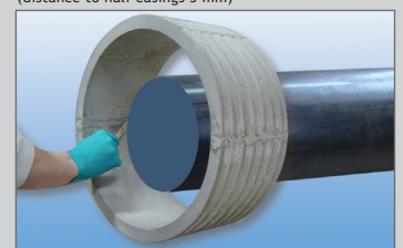
Distribute filler evenly so that the inner surface forms a homogeneous seal surface, smooth with emery cloth, if necessary
