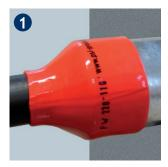
Pull sleeve over the carrier pipe and the casing pipe. The edge of the casing pipe should be chamfered.
