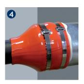
Then install the second strap. Spread leaking adhesive, if necessary.
