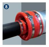
Finally, the sleeve has to be protected by means of an expansion pad.
