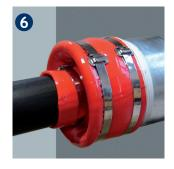
Align the sleeve on the carrier pipe elongated (figure a) or S-shaped (figure b) depending on the extension direction. Then install the first strap about 15 mm away from the rear end.
