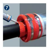
Inject the adhesive underneath the sleeve the way you did with the casing pipe side and install the second strap. Spread leaking adhesive, if necessary.
